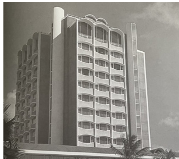
Figure 30 - Tower as part of the expansion (source: Fischer)
