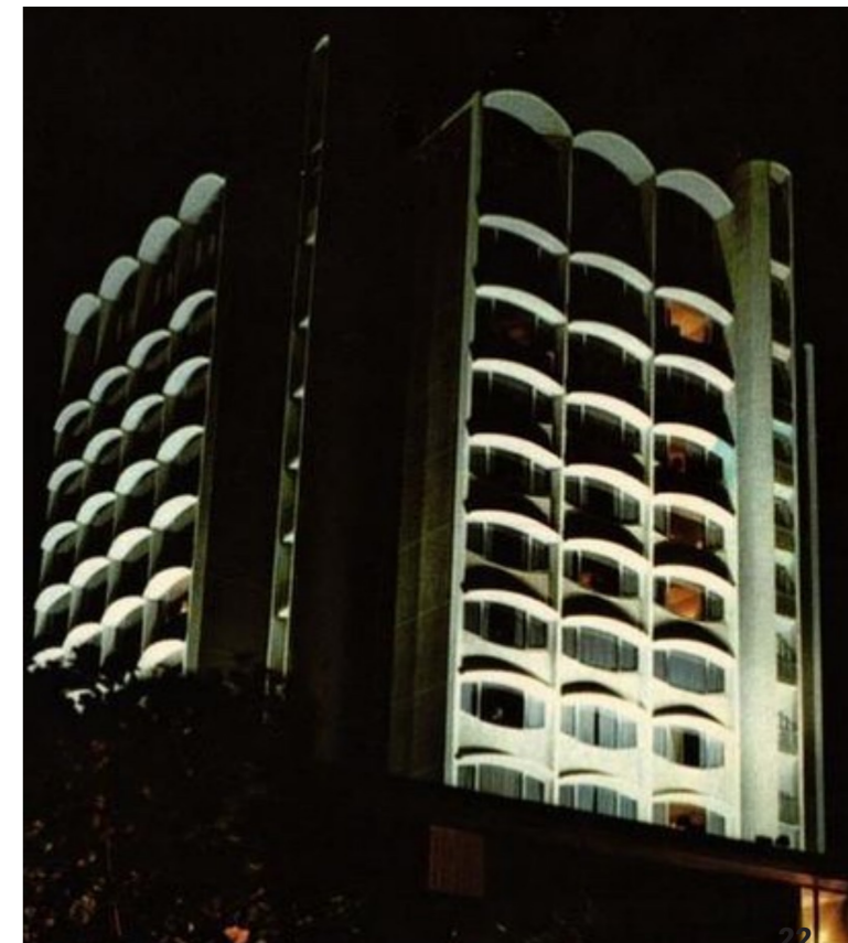
Figure 32- Tower illuminated at night (source: Curacao archive)
