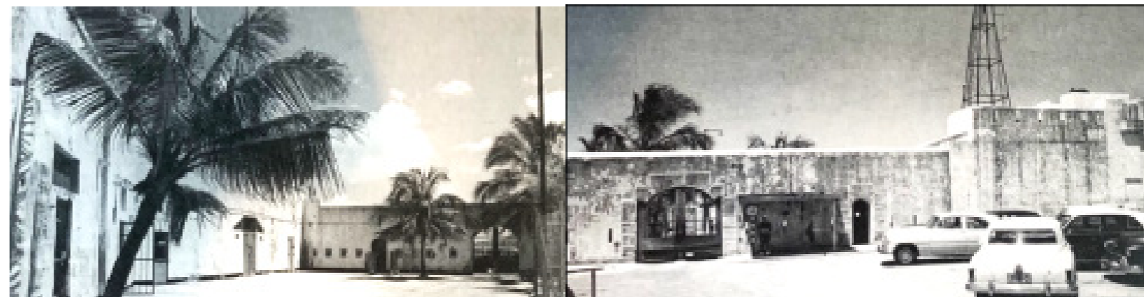
Figure 37. The entrance of The Waterfort from the inside (left) and outside (right). The entrance wall was removed in 1955 (Hartog, 1997)
